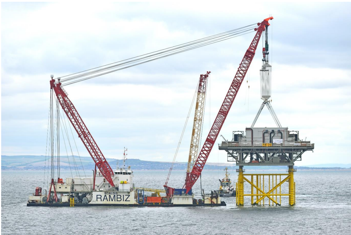
Graphic 4-11 Example offshore substation during installation (Rampion 1 offshore wind farm)
