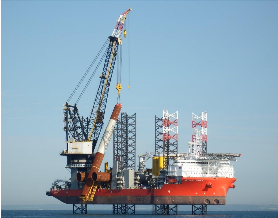
Graphic 4-8 Example JUV installing a WTG monopile foundation (Rampion 1 offshore wind farm)
